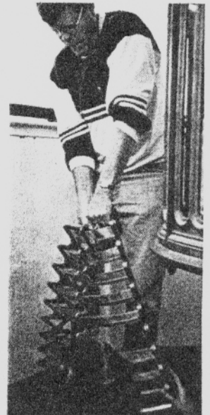
Bob Llewellyn removes an upper section of the lens from the lantern room.
