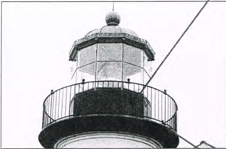
LANTERN ROOM AND GALLERY DECK
