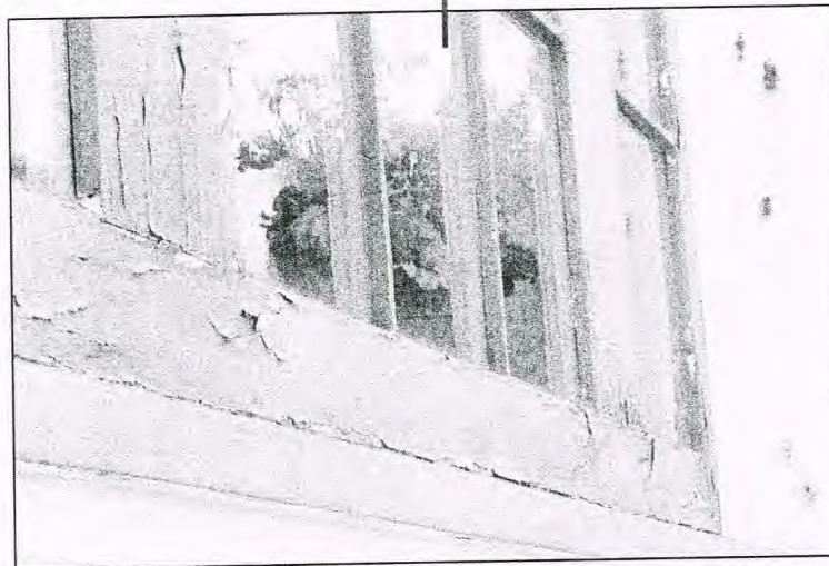
DETERIORATING WINDOW CONDITION DUE TO PEELING PAINT AND RUST
