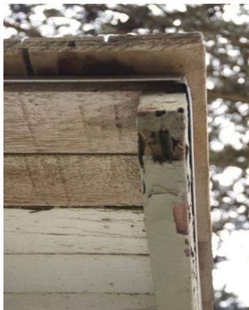
Figure #52: Example of wood rot on rafter tail.
