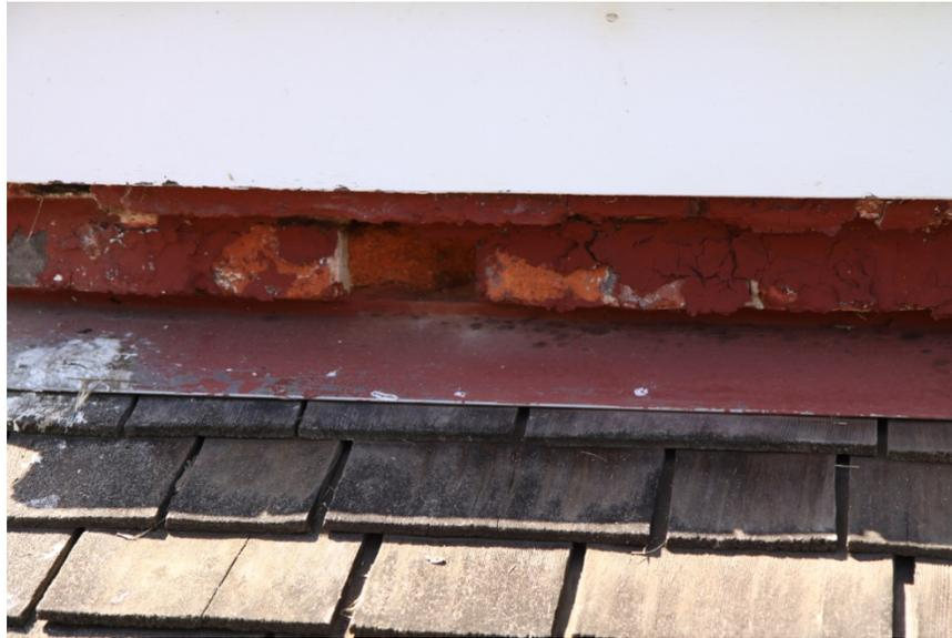
Figure #40: TYPICAL CONDITION OF BRICK CORBEL-**POOR**.
