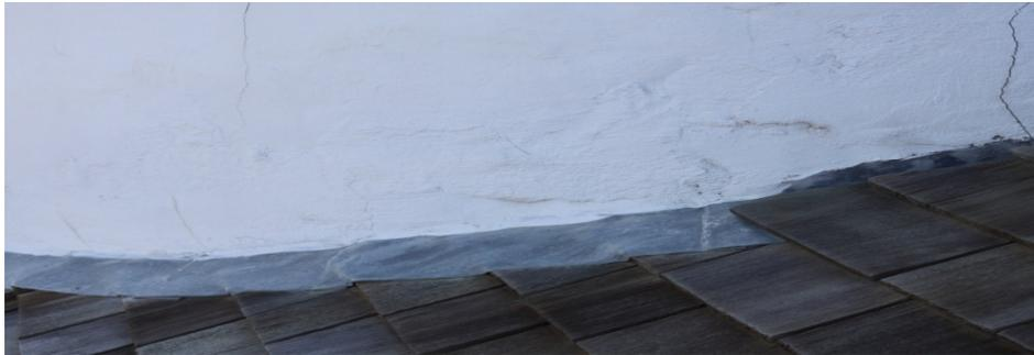
**Figure 5: Example of failed stucco coat with resultant loss of protection and additional moisture entry behind stucco coat. Crack allows avenue for water behind metal flashing and into interior walls.**
