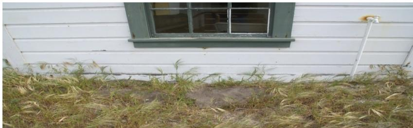
Figure 18: Accumulated dirt and vegetation should be raked away from contact with wood ASAP.
