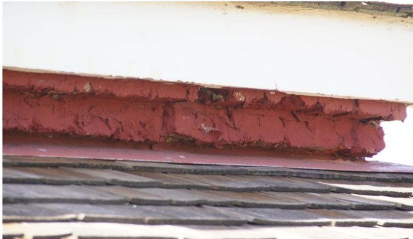
Figure #41: TYPICAL CONDITION OF BRICK CORBEL-**POOR**
