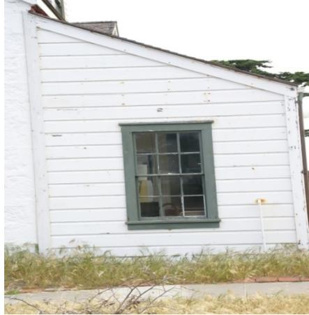
Figure #21: 6/6 DOUBLE HUNG WINDOW -REAR ATTACHMENT-**POOR**.
