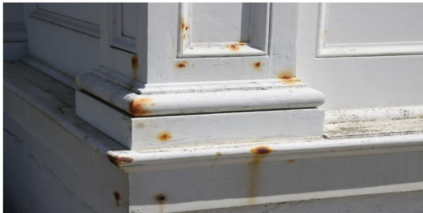
There is a high degree of decorative fenestration on the front porch of the lighthouse. The fenestration has been rated as **FAIR** to **POOR**. There is widespread oxidation stains and loss of protective coatings. These conditions could be repaired by volunteers to reduce City of Pacific Grove cost.
