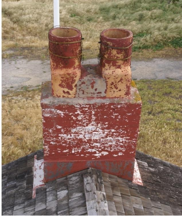
Figure #39: TYPICAL EXISTING CONDITION OF HISTORIC CHIMNEY SYSTEM.
