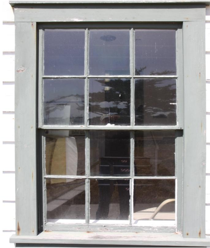
Figure#28 : TYPICAL WINDOW CONDITION-POOR
