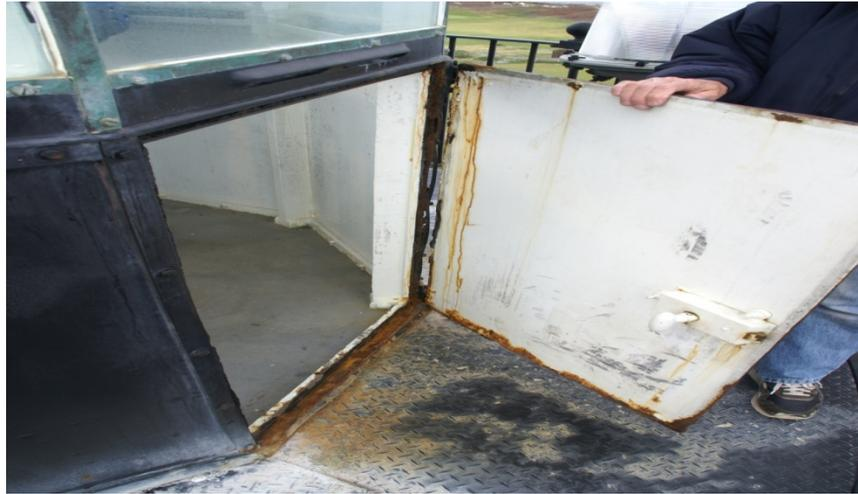
Figure#10: Inside surface of Lantern Room door requires immediate and extensive repair.
