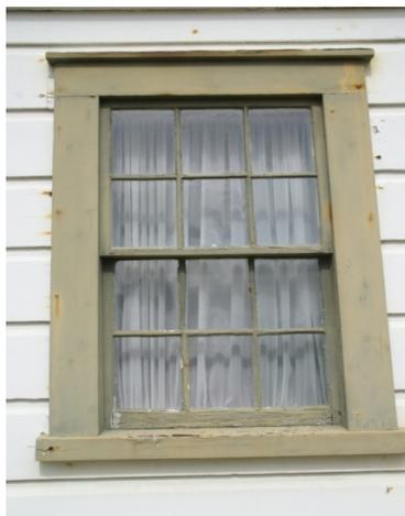
Figure# 16 & 17: 6/6 DOUBLE HUNG SASH
