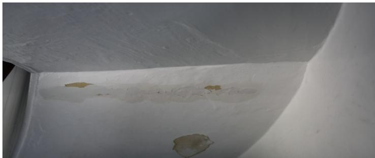
Figure :Moisture stains on inside of lantern support cylinder/stairwell.
