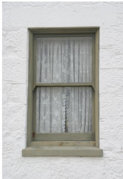
Figure #10: WEST ELEVATION-WINDOW- FAIR to **POOR**.
