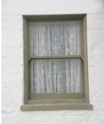
Figure #9-WEST ELEVATION WINDOW-GOOD to FAIR.
