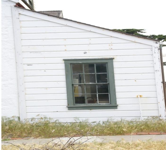
Figure : Build up of earth and vegetation against wood fabric.
