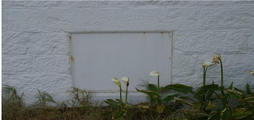
Figure #8: ENCLOSED BASEMENT WINDOW-NORTH-POOR.
