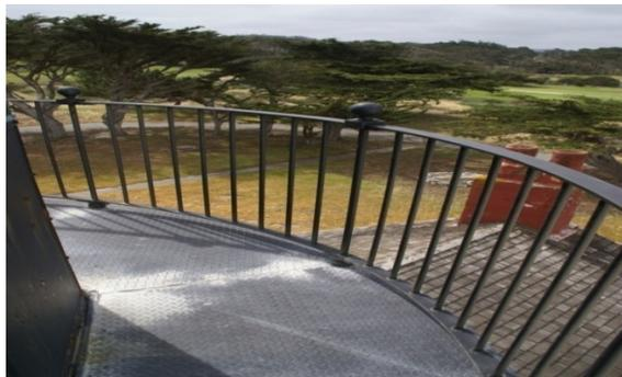
Figure 8: Textured deck plates. Note oxidation of surface.
