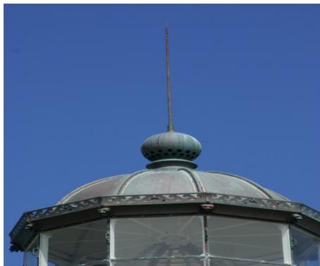
Figure 7 : Lightning rod and vent ball.
