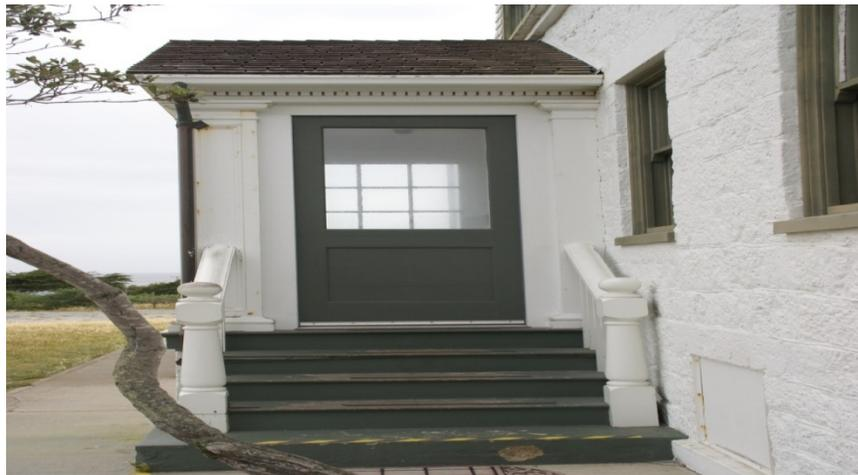
The entrance steps have been rated **FAIR** to **POOR**. There are small areas of spalled concrete requiring patchwork to prevent additional damage and moisture entry.
