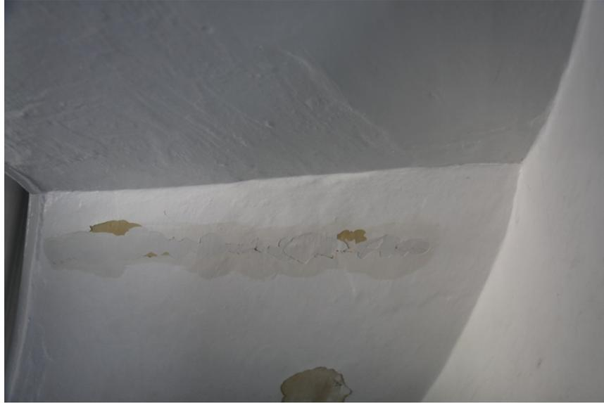
Figure3: Evidence of moisture damage from exterior cracks in stucco.
