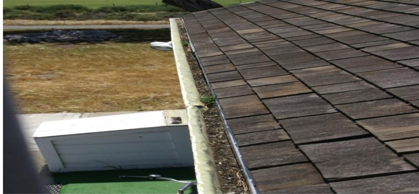
Figure: Gutters filled with debris.
