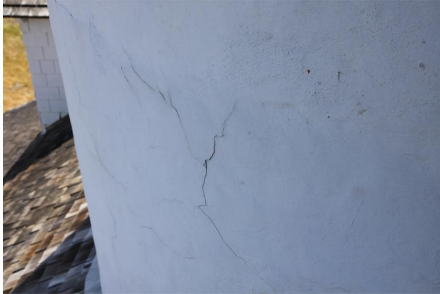
Figure 3: Cracks in stucco.
