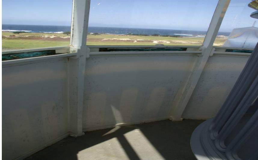
Figure #5: FLAT IRON LANTERN ROOM WALL PANELS.
