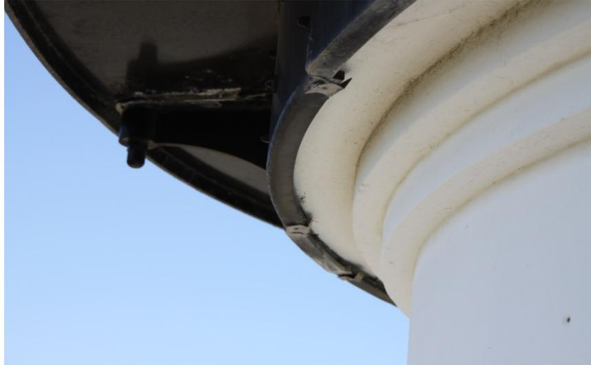
Figure 9: Brick corbel serves as part of lantern room support system.
