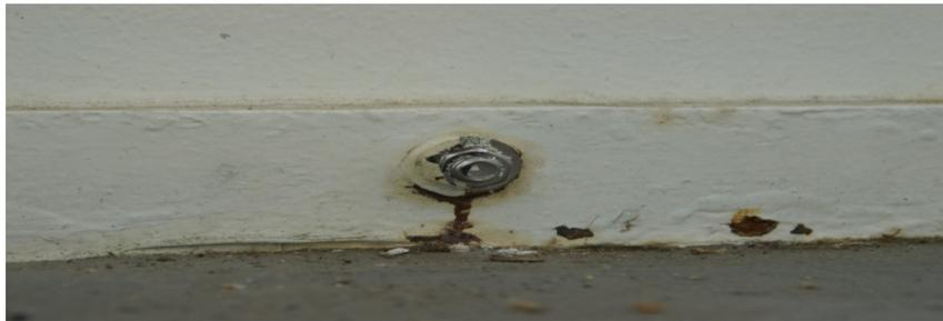
Figure #9: Stainless steel fasteners used to attach exterior flashing.
