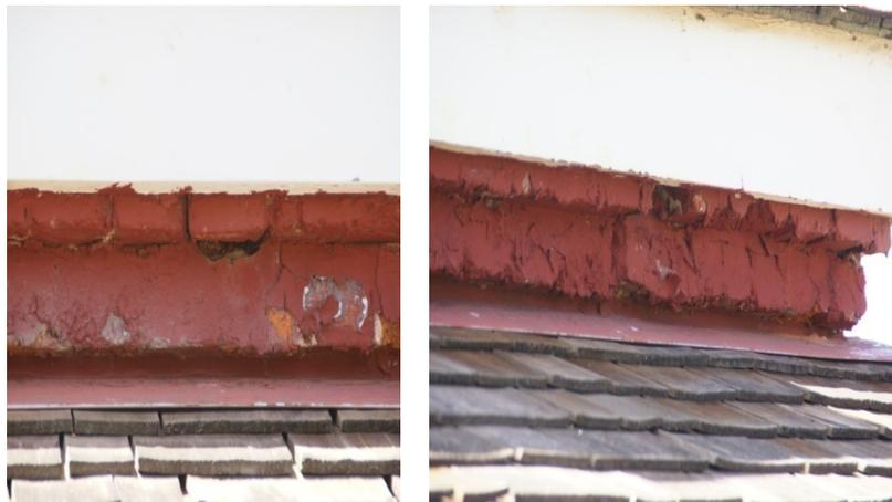
Figure 29 & 30: Examples of type of damage to roof brick corbel.
