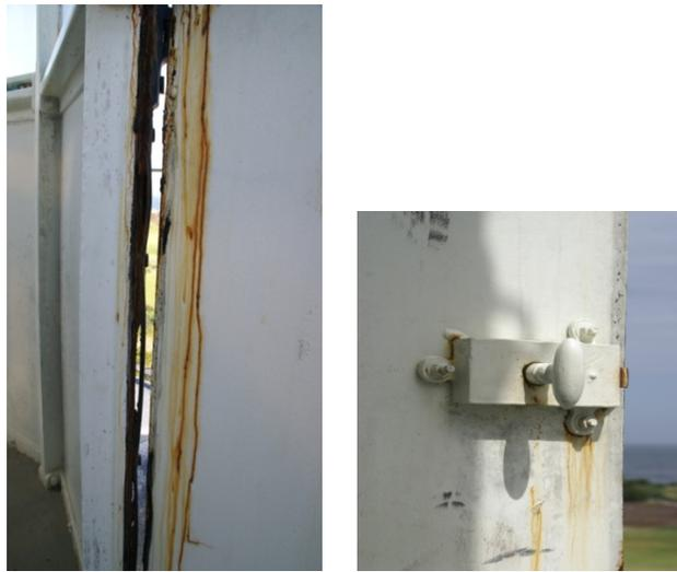
Figure# 11 & #12: Historic lock mechanism must be preserved and used.
