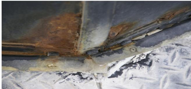
Figure: Damage to deck plate and aluminum flashing.
