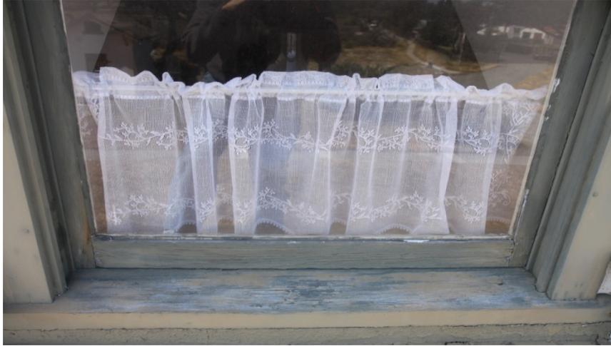
Figure # 30: LOSS OF PROTECTIVE COATINGS -WINDOW SILL-**POOR**
