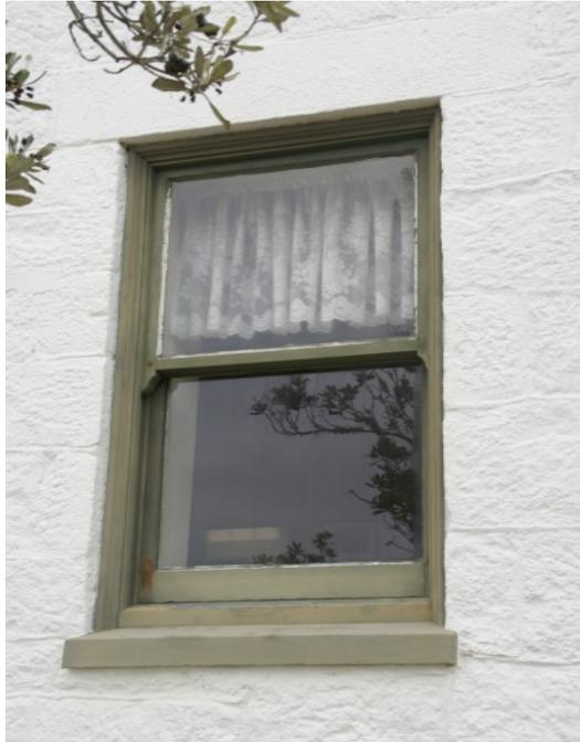
Figure #1.1/1 DOUBLE HUNG SASH WINDOW WEST ELEVATION **GOOD** to **FAIR**.
