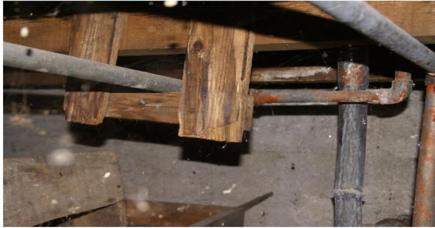
Figure #24: Leaking water pipe below bathroom.
