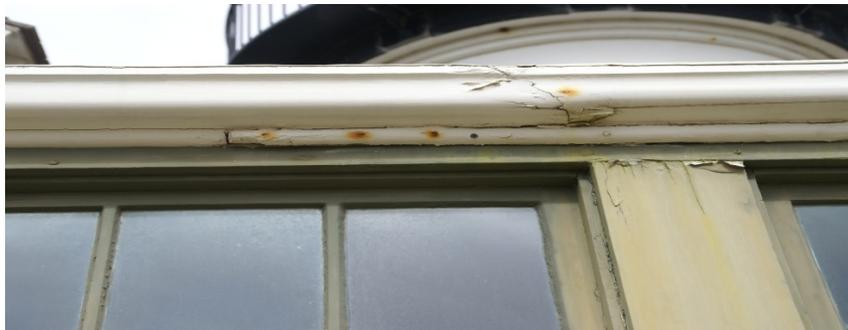
Figure: Gutter system has numerous areas of damage related to failed fasteners.
