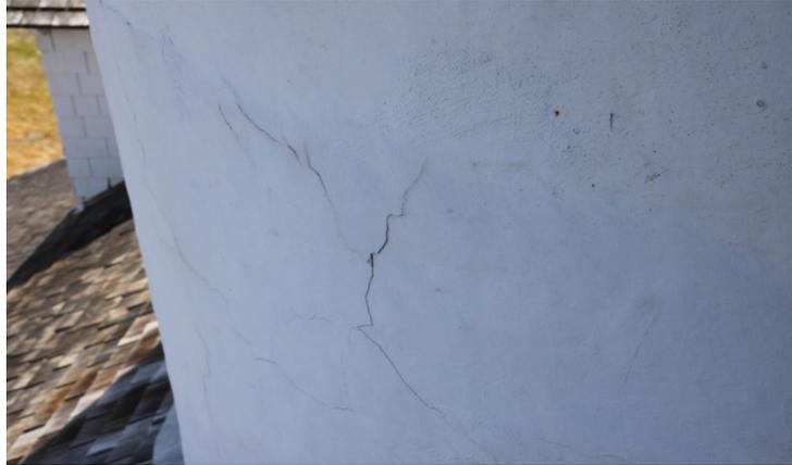
Figure : LANTERN ROOM SUPPORT CYLINDER
