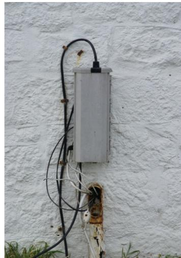
Figure 20 & 21: Obsolete equipment and attachments should be removed and historic fabric repaired.
