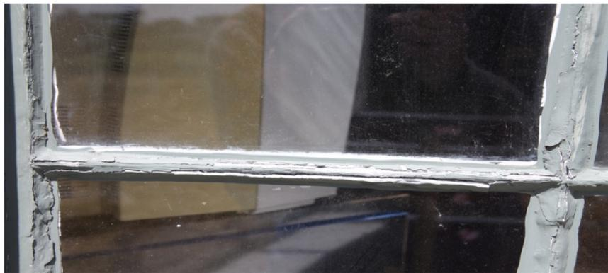
Figure #29: LOSS OF WINDOW GLAZING-POOR
