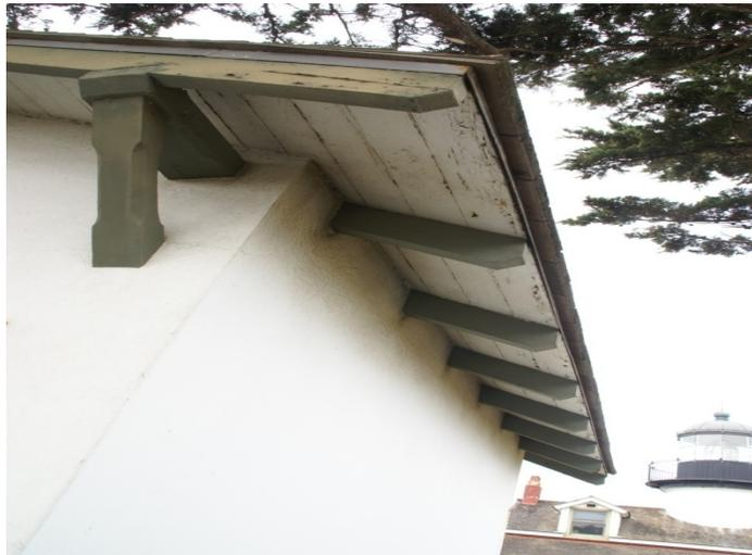
Figure #54: Example of severe crack in fascia board.
