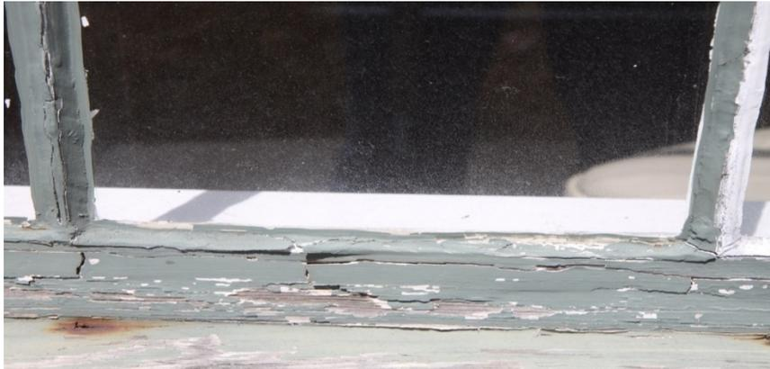
Figure #31: LOSS OF PROTECTIVE COATINGS WINDOW SASH-**POOR**
