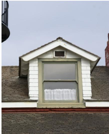
Figure #14: DORMER WINDOW EAST ELEVATION-FAIR to **POOR**.
