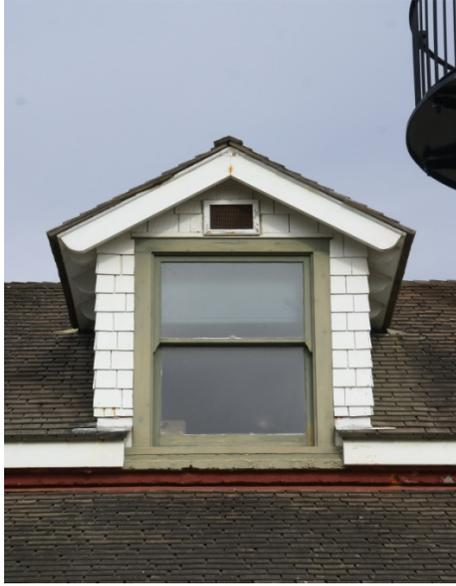
Figure #13: EAST ELEVATION DORMER WINDOWS-FAIR to **POOR**.
