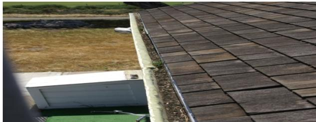
Figure 23: Roof gutters and downspouts should be cleaned ASAP.
