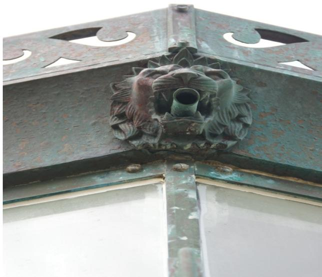
Figure: Bronze Lion Head gutter/downspout
