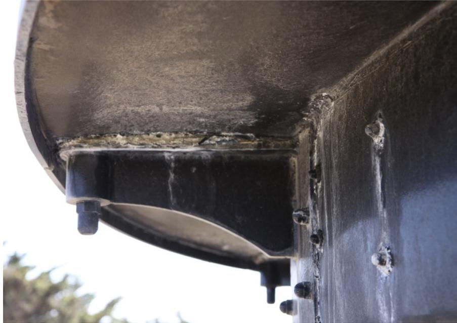
**Note missing nut on far right support bracket. Note build up of aluminum oxide along top edge of bracket along seams and connector bolt heads.**
