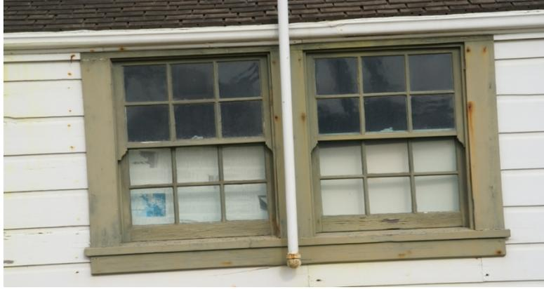
Figure#15 : EAST ELEVATION WINDOWS 6/6 double hung sash windows.-**POOR.**
