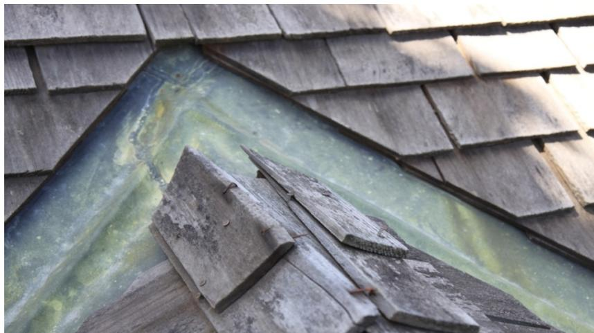
Figure #45 : RIDGE CAP DORMERS-NOTE MISSING RIDGE CAP.
