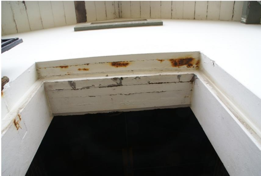
Figure #58 & #59: Typical conditions of iron door frame.
